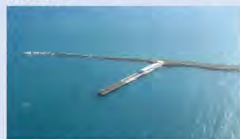
Figure 4. Aerial photo of Rompeolas (Mosquito Pier) at Vieques, PR.
